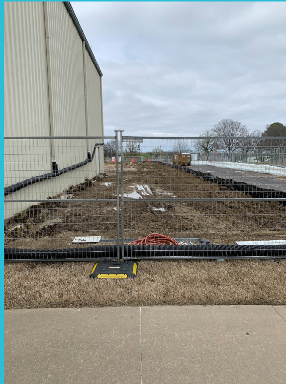
Temporary Roof Drainage
