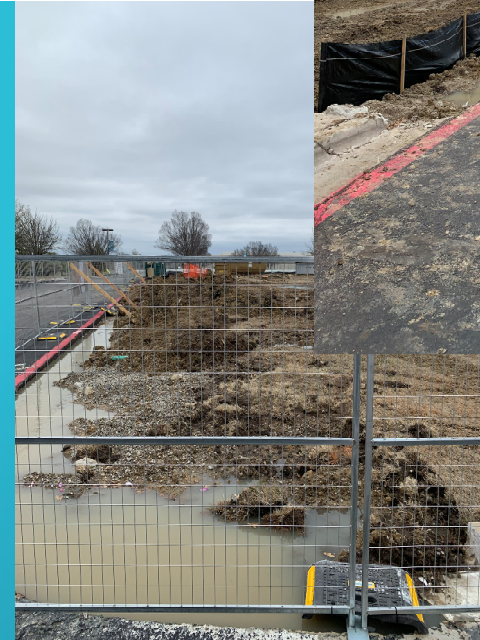
Silt Fence Installation
