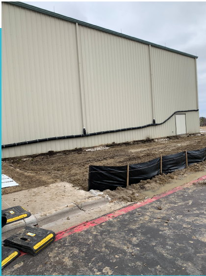
Temporary Roof Drainage
