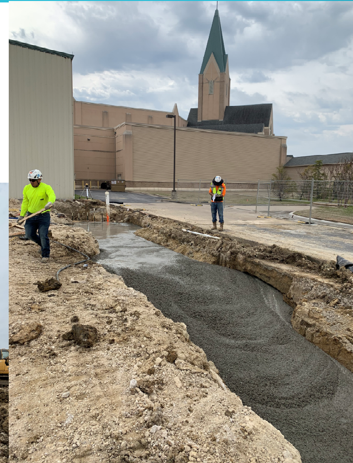
Footing Excavation and backfill
