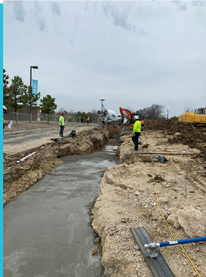
Footing Excavation and backfill
