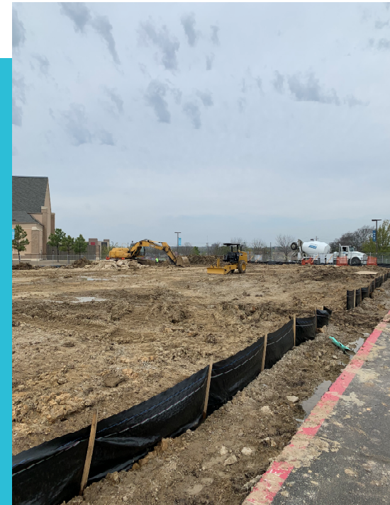
Building Pad and Silt Fence
