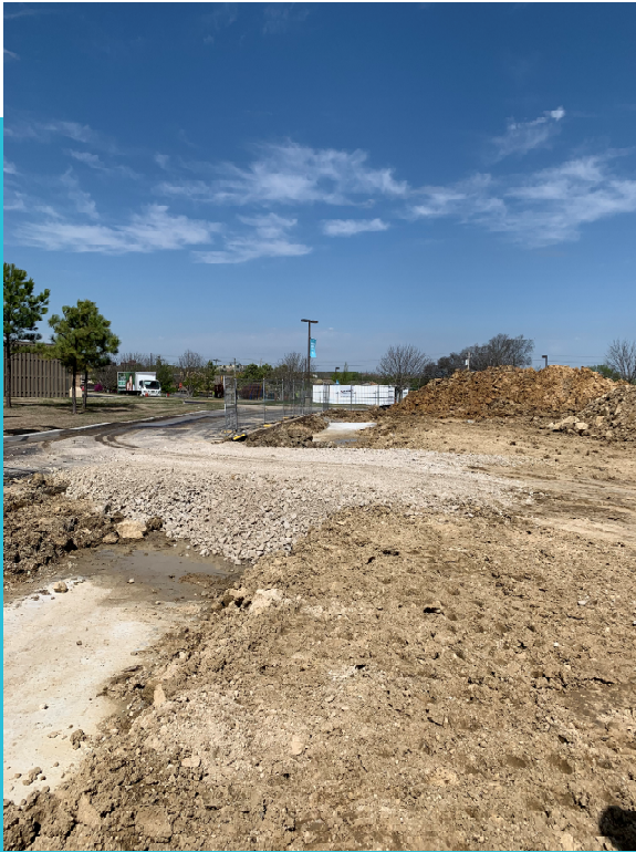
Temporary Road over Footing Excavation
