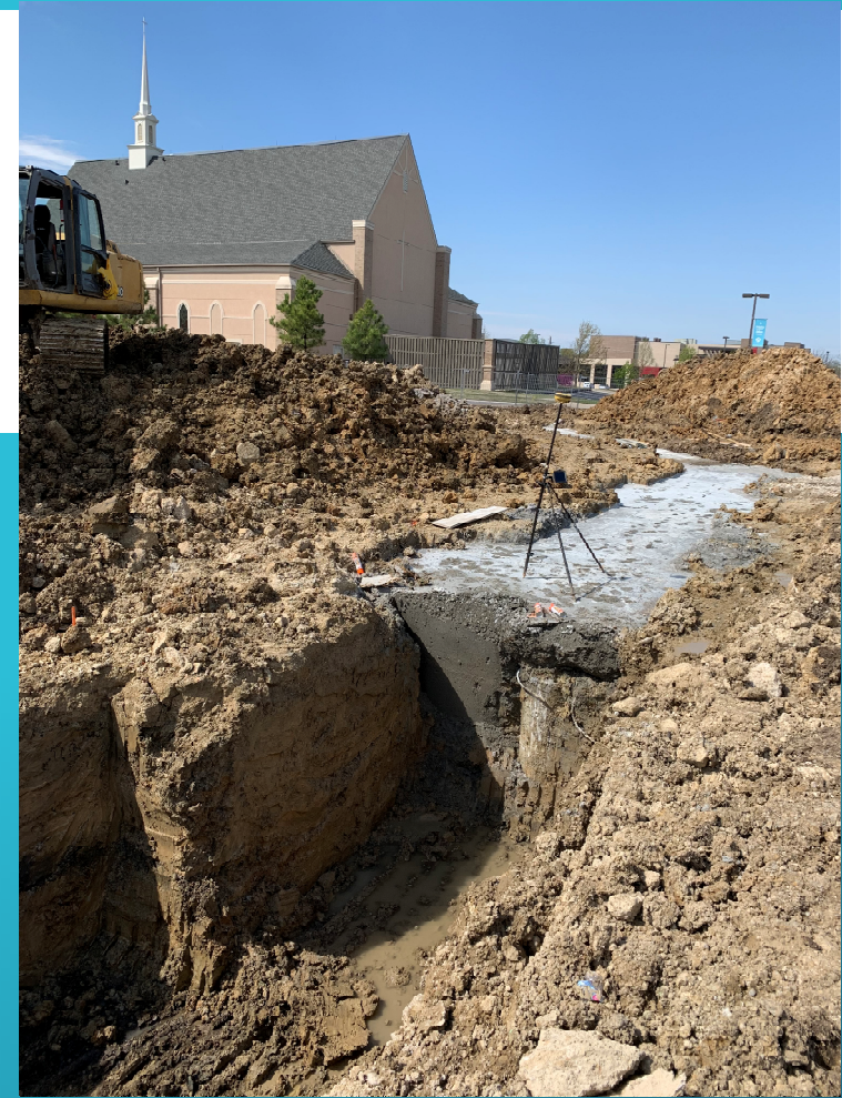
Footing excavation and backfill continue
