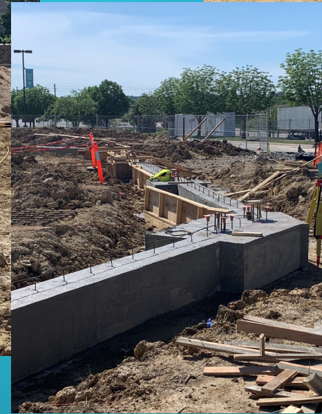
Footings partially complete
