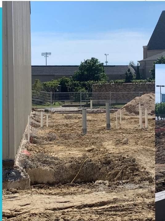
Under slab electrical & plumbing rough-in
