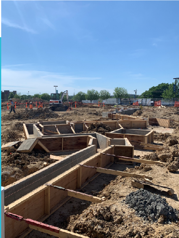
Concrete footing layout and forming continues
