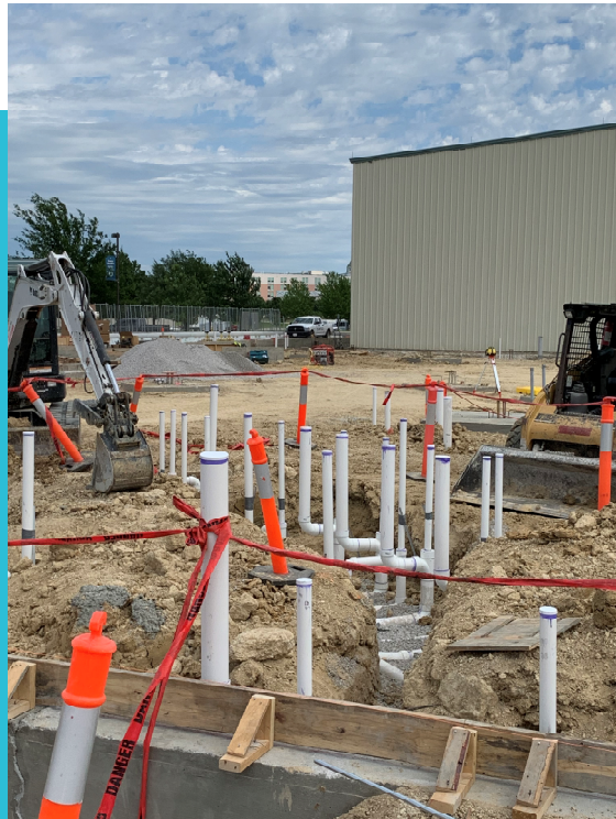
Under slab plumbing rough-in at Restrooms
