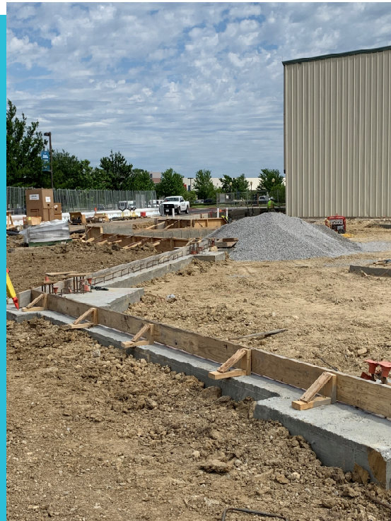
Slab edge forms are being installed
