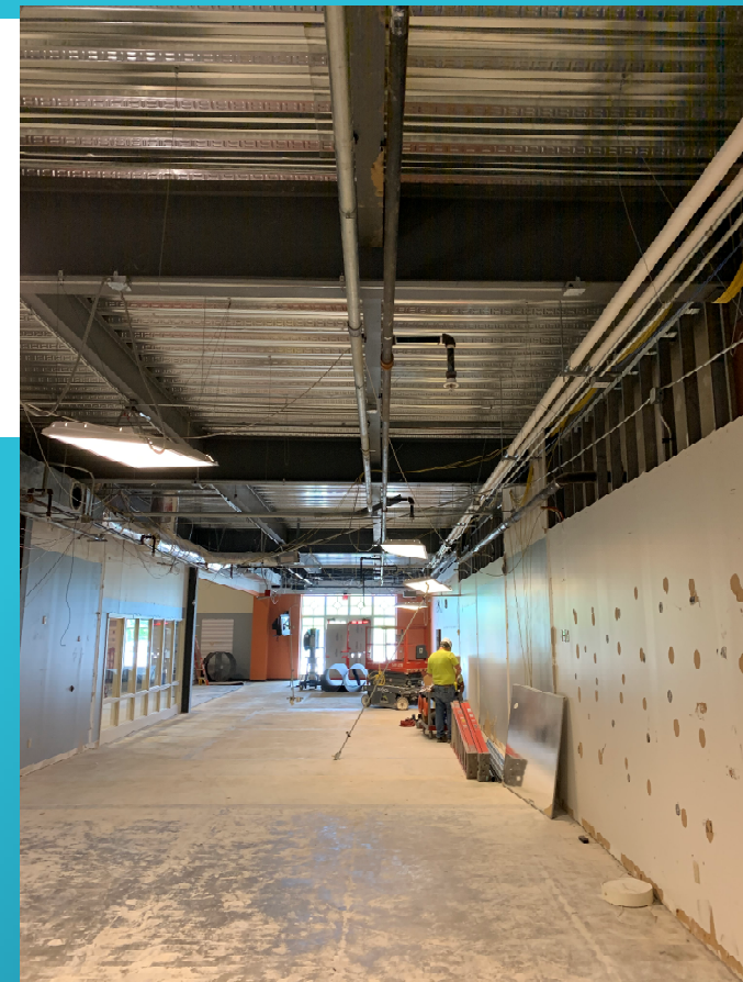
Gym Demolition has started
