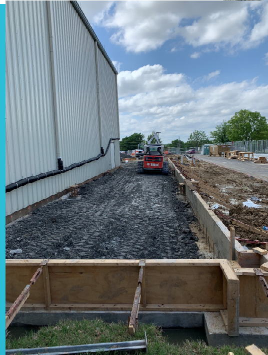
Slab edge forms installed and building pad set to grade
