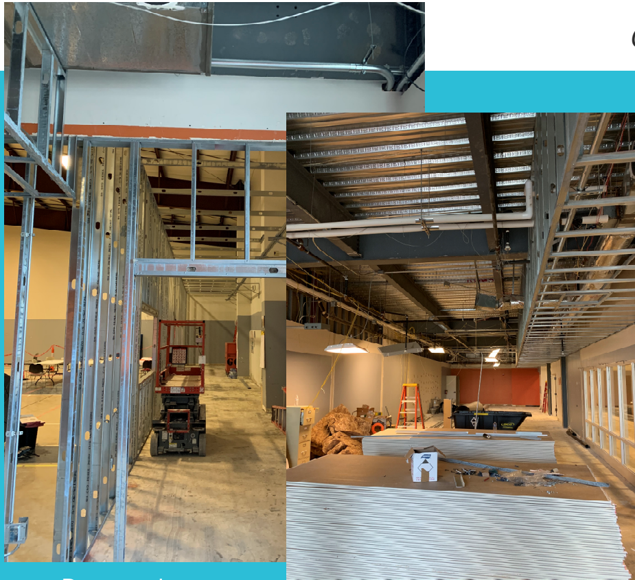
Renovation – Student Commons Center wall Framing
