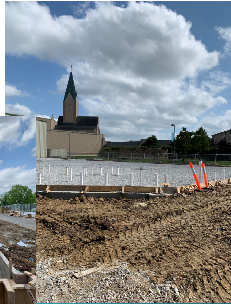
Building Slab Ready for Rebar
