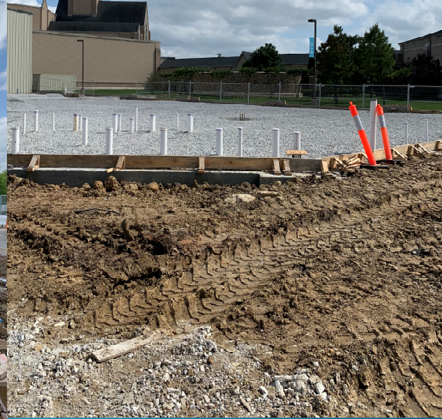
Building Slab Ready for Rebar
