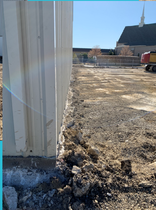
Site demolition complete adjacent to gym
