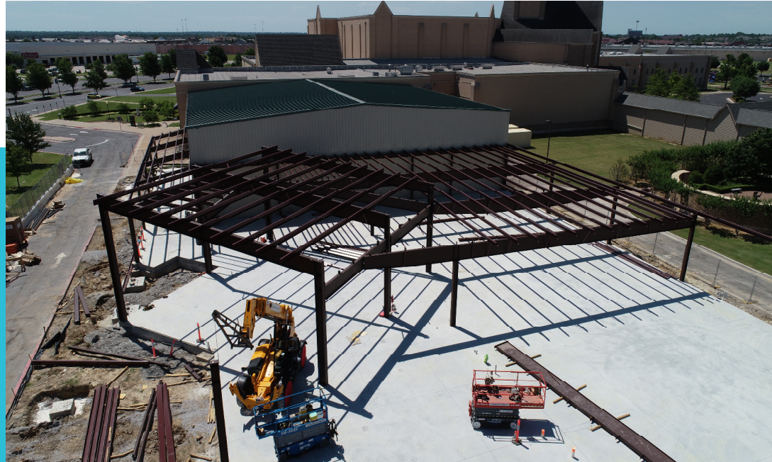
Building Steel erection is taking shape
