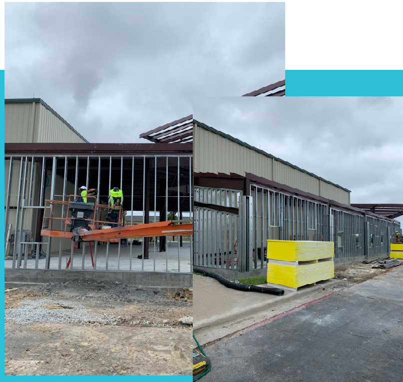
Exterior Wall Framing and Sheathing
