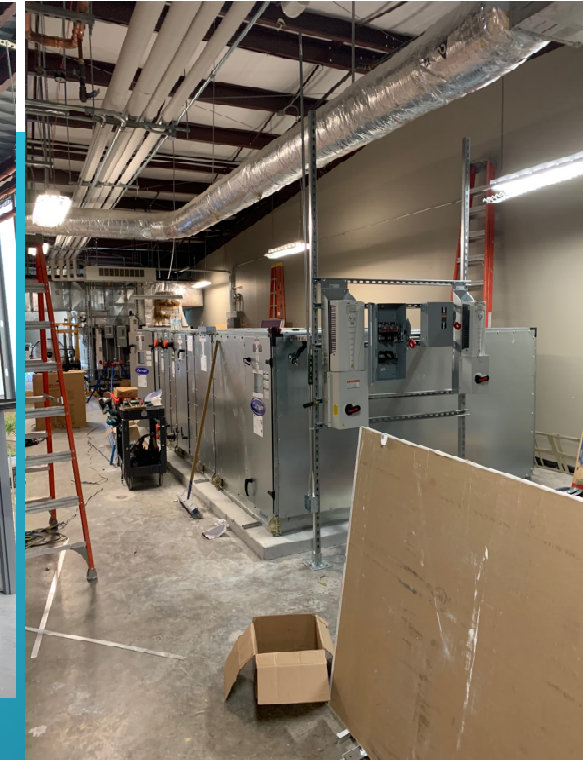
Renovation: HVAC unit is being hooked up
