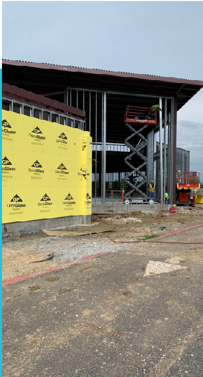
Exterior Wall Framing and Sheathing Continue
