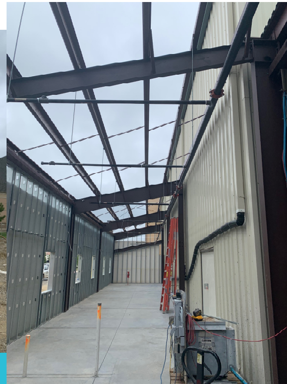
Overhead Fire Protection rough in & Wall layout at offices
