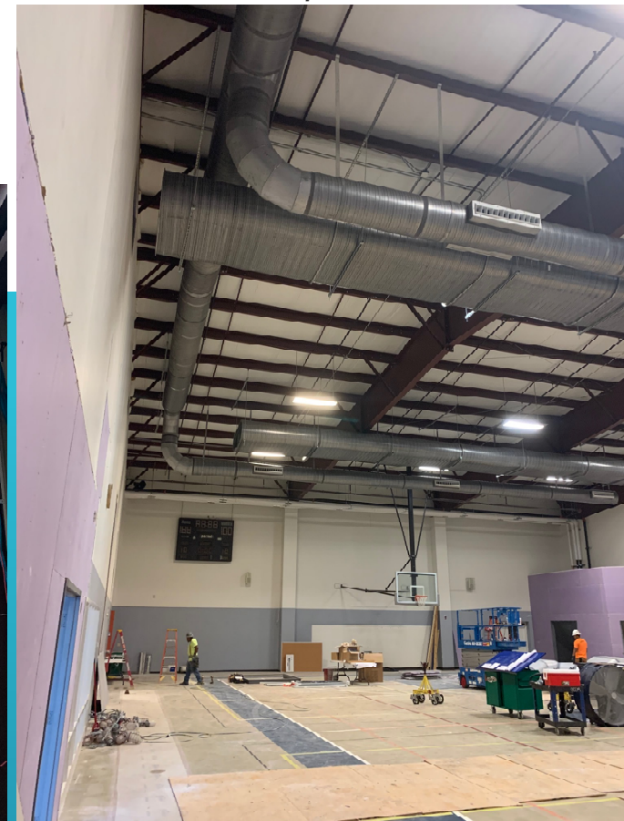
Renovation: Gym Duct work and New Addition Supply Duct work
