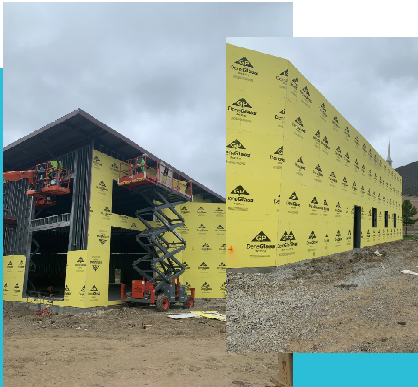
Exterior Wall Framing and Sheathing Continue
