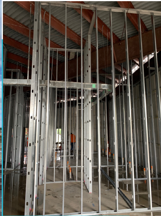
Interior wall frame and door jambs are being set
