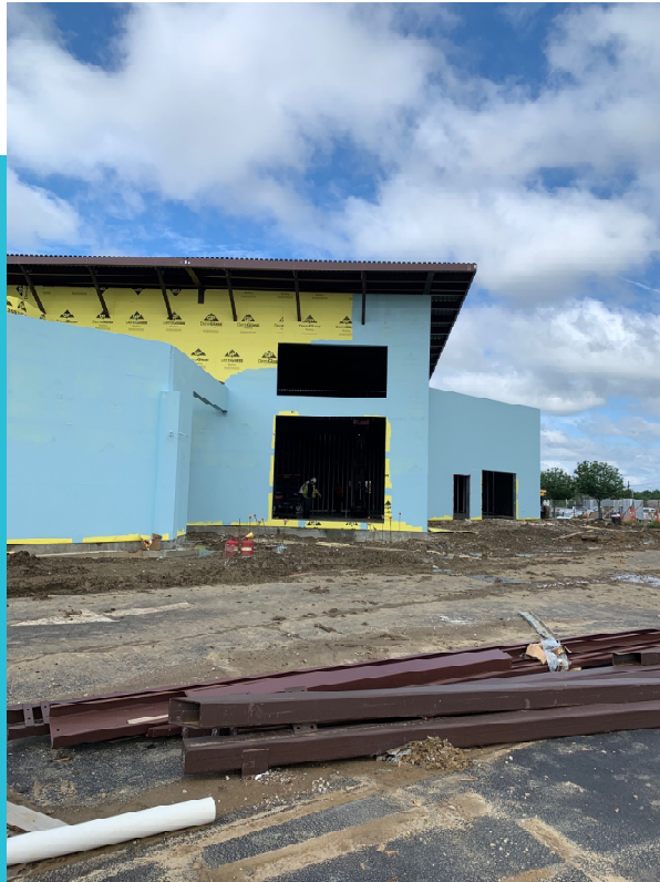
Vapor barrier is being installed
