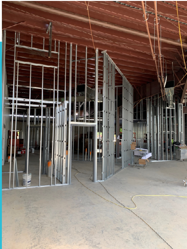
Interior wall framing continues
