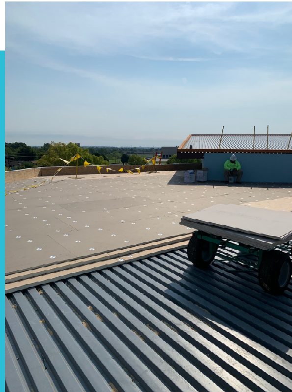
Roofing has started
