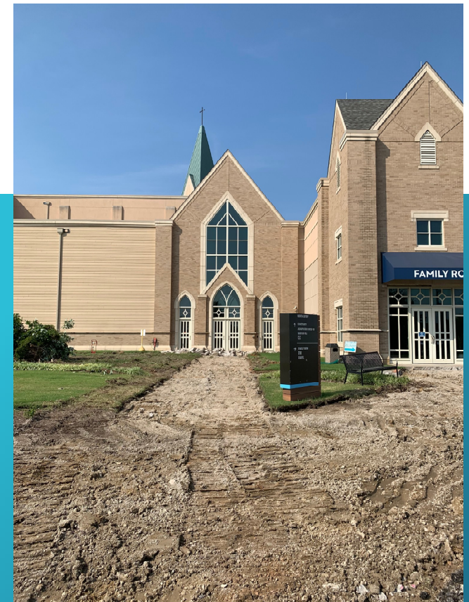
North Portico – Demolition has started
