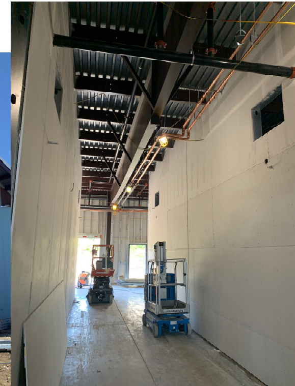
Sheetrock Installation
