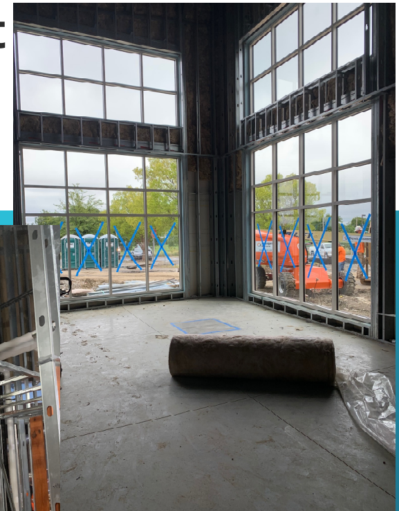
Ceiling Framing and Glass Installation
