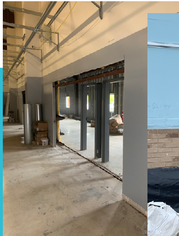
Existing Building is not connected
