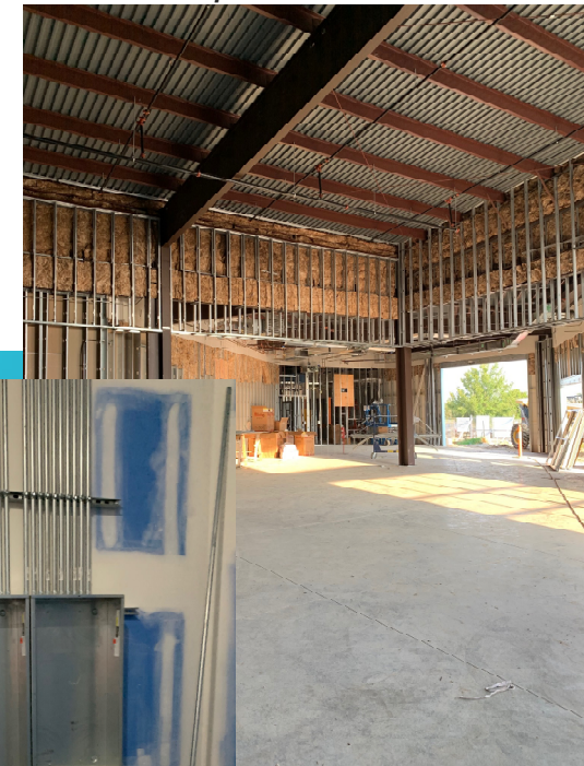
Electrical panel boxes and wall rough in
