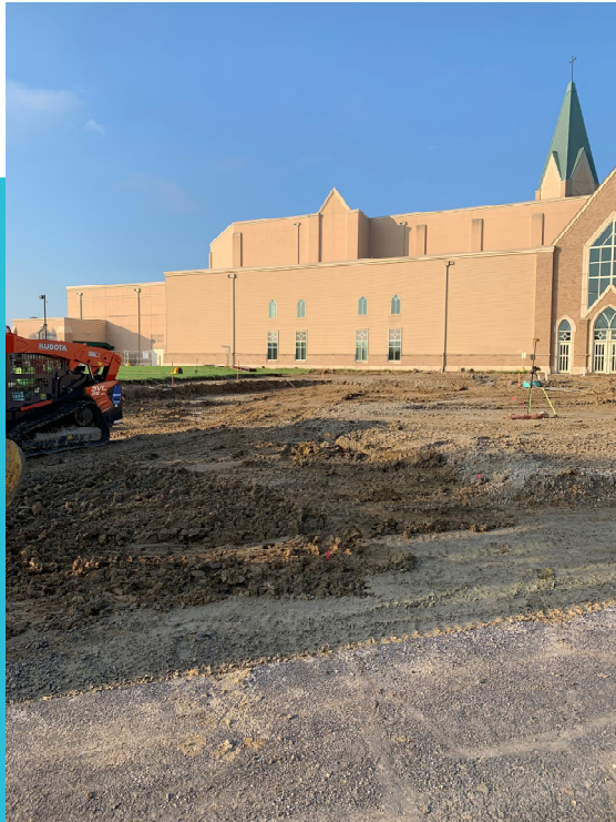
North Portico Grading Continues
