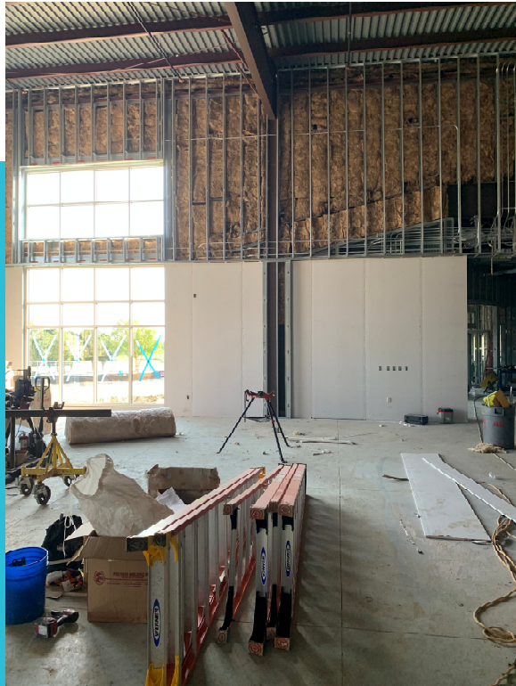
Sheetrock installation
