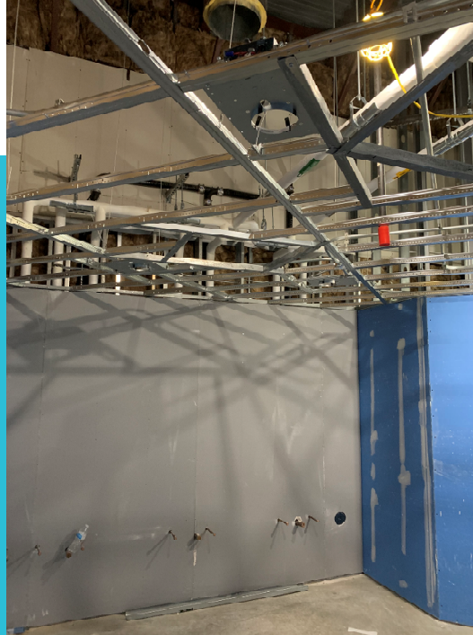
Above ceiling rough in for lighting
