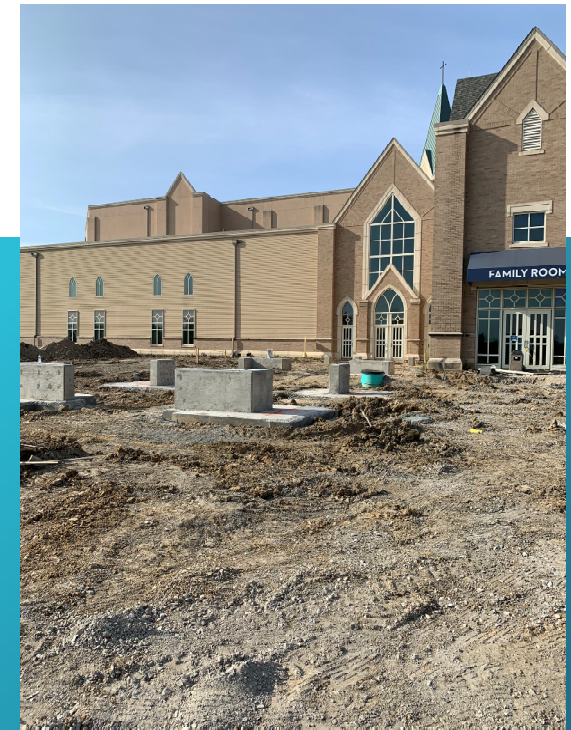
North Portico foundations ready for steel
